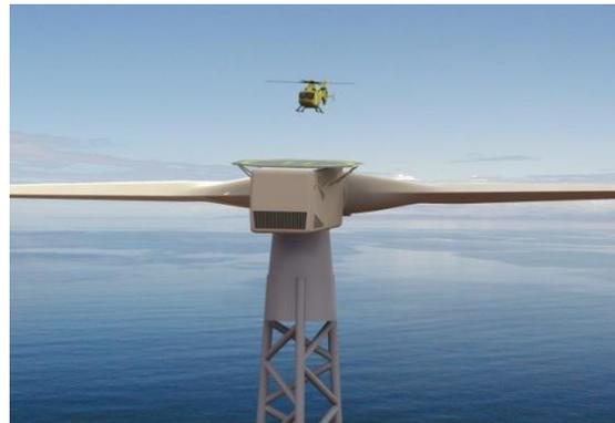
Figure 9: 2-blade offshore wind turbine (2B Energy)
