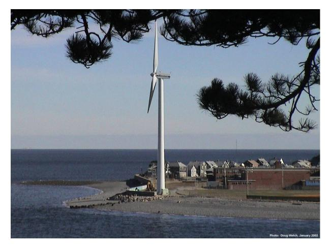
Hull Wind I, Hull, MA, Vestas 660 kW, 47 m diameter, 50 m tower; 2001
